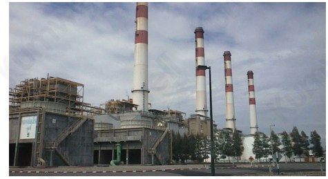
THAILAND : PTT GASSEPARATION PLANT
